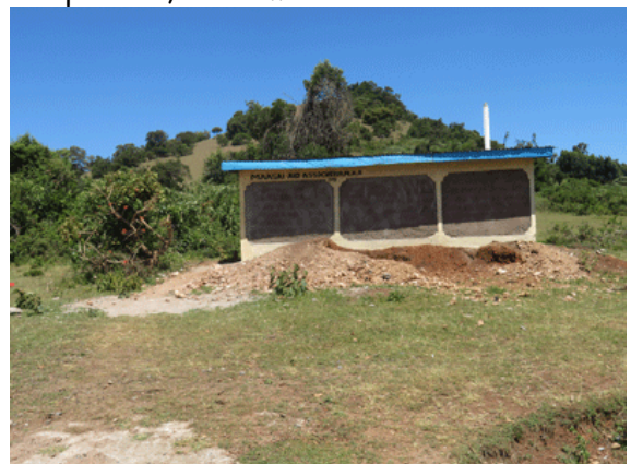
The 6 new latrines, necessary after increasing the number of school classes.
